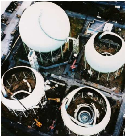
Gas holders (apple peeling method)
